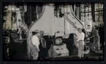
**1929** - Continuing to solve customers tooling problems while building on their expertise in supplying specialty steel open die forgings, Anderson Shumaker installs a new 6,000 pound hammer.
